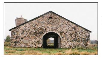
In the early 1990's the north wall began to lean outward causing many cracks in the structure, threatening the walls to collapse.
