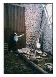
Some of the cracks were very large and detrimental to the structure.
