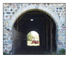
The barn was designed with two large arched doorways so you could enter through one end with a wagon full of loose hay, unload the hay into the loft, and then drive out the other end.
