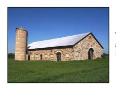
The barn measures 100 feet long by 60 feet wide. The walls are two feet thick and are estimated to weigh 2 tons per linier foot.
