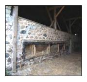
Another unique feature of the barn is the half stone wall that separates the threshing area from the stable area. It was also used as a porthole to pass feed through. Feed was dropped over the edge of the loft and then pushed by hand through the wooden hinged doors into the stable area on the other side.
