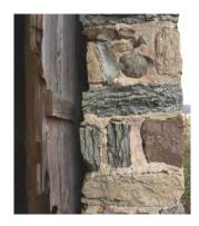
The walls of the barn were built entirely of stone and lime putty mortar. Many types of stones were used including granite, quartz, mica, feldspar, gneiss, hornblende, gabbro, and schist. Some of the stones are over two billion years old!
